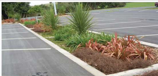
Use of native plants within landscape areas of parking lots can aid in removal of contaminants and sediments from stormwater prior to drainage into the watershed.
