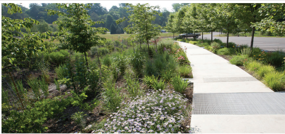
Bioswales, similar to drainage ditches, utilize selected vegetation to filter and slow down stormwater runoff prior to its drainage into the water shed. These bioswales can be designed using native vegetation adapted to the area, requiring minimal maintenance.
